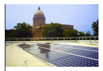
Frankfort's new Visitors Center now has an array of solar panels on its roof that will supply supplemental green energy to the building. The installation consists of 24 photovoltaic, self-ballasted modules. The light weight modules are designed for a flat roof application and are tilted 10 degrees to better catch sunlight and shed dirt and rain. Each module can generate up to 305 watts of power. The total array can produce up to 8,000 kWh each year.
